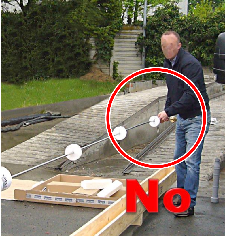
Attention: The probes must not be bended!
