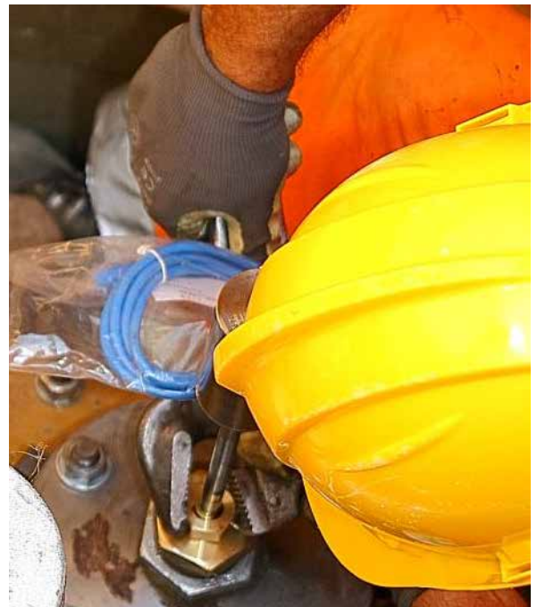
Tighten the gland bolt at this "Safety Distance"
