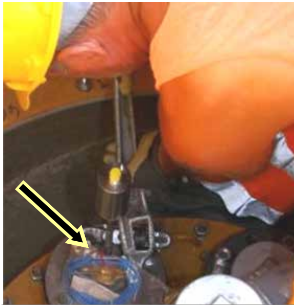
Screw the screw-in unit into the flange (resp. reducer)
