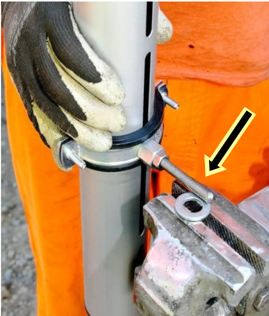
Mounting example with washer welding by installer
