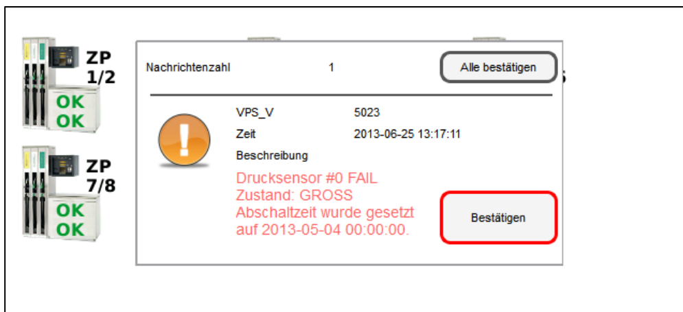
Alarms and Shutdown of SECON-Client (series of pictures)
